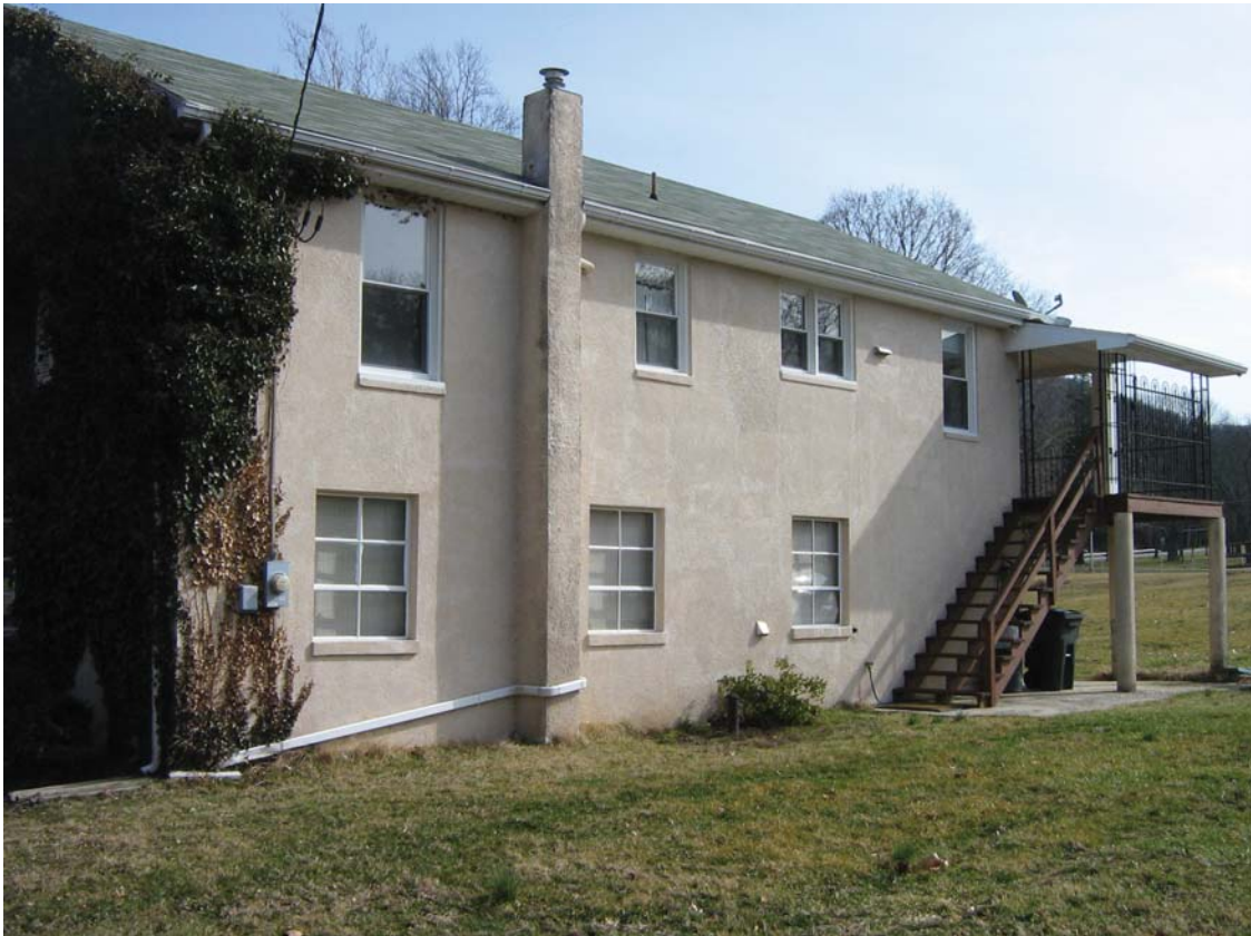
Rear of residence at 5 Willow Road
