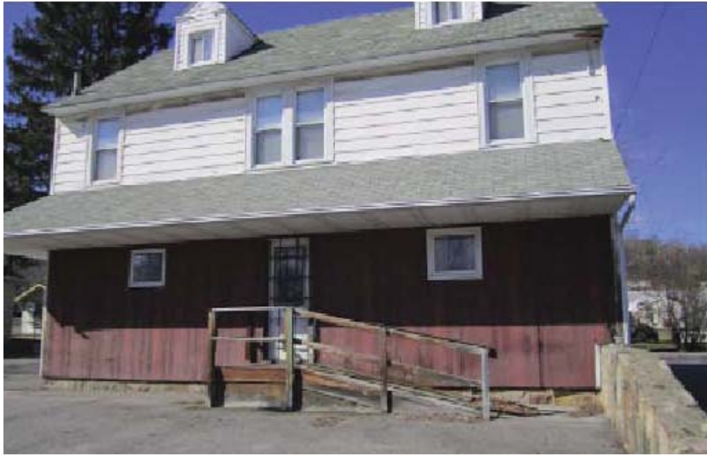
Front of residence at 226 -230 E. Wopsonnock Avenue
