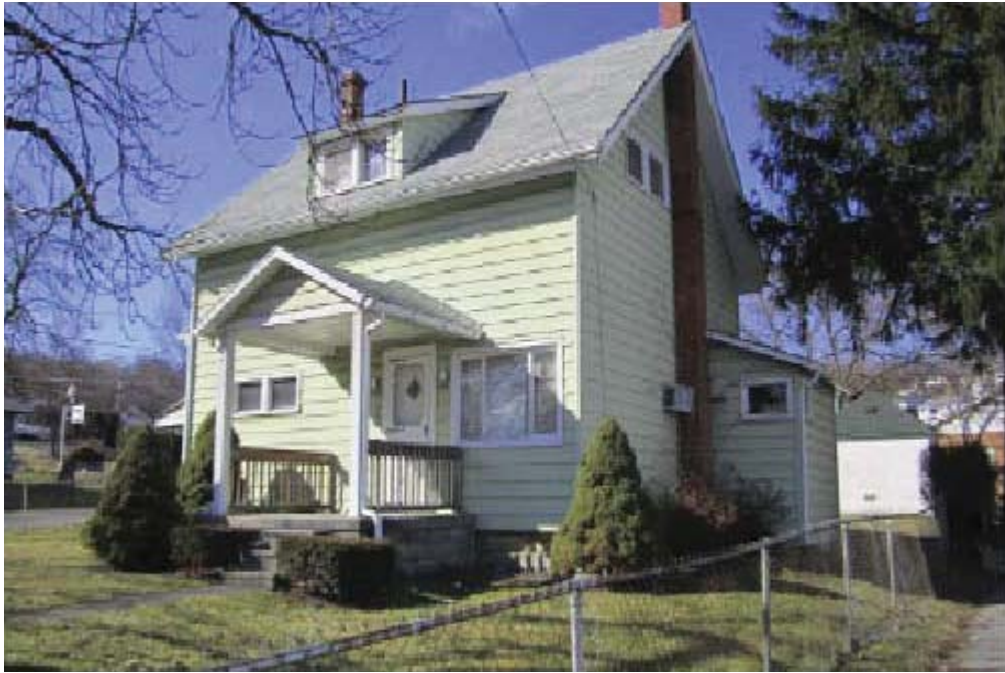
Front of residence at 226 -230 E. Wopsonnock Avenue
