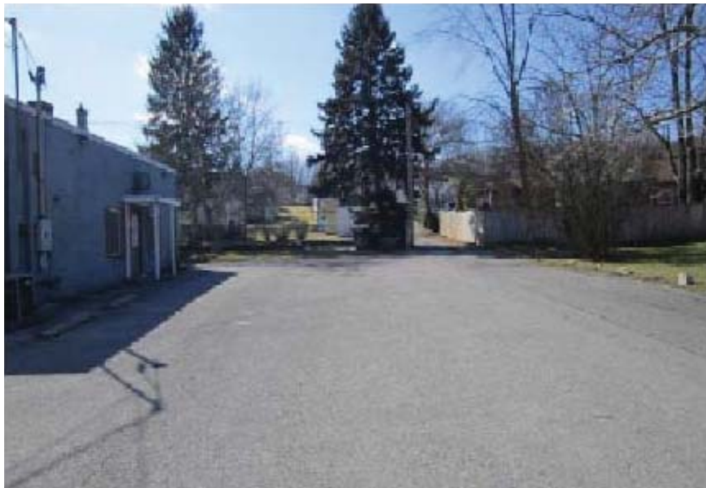
Rear of commercial building at 232 -236 E. Wopsonnock Avenue
