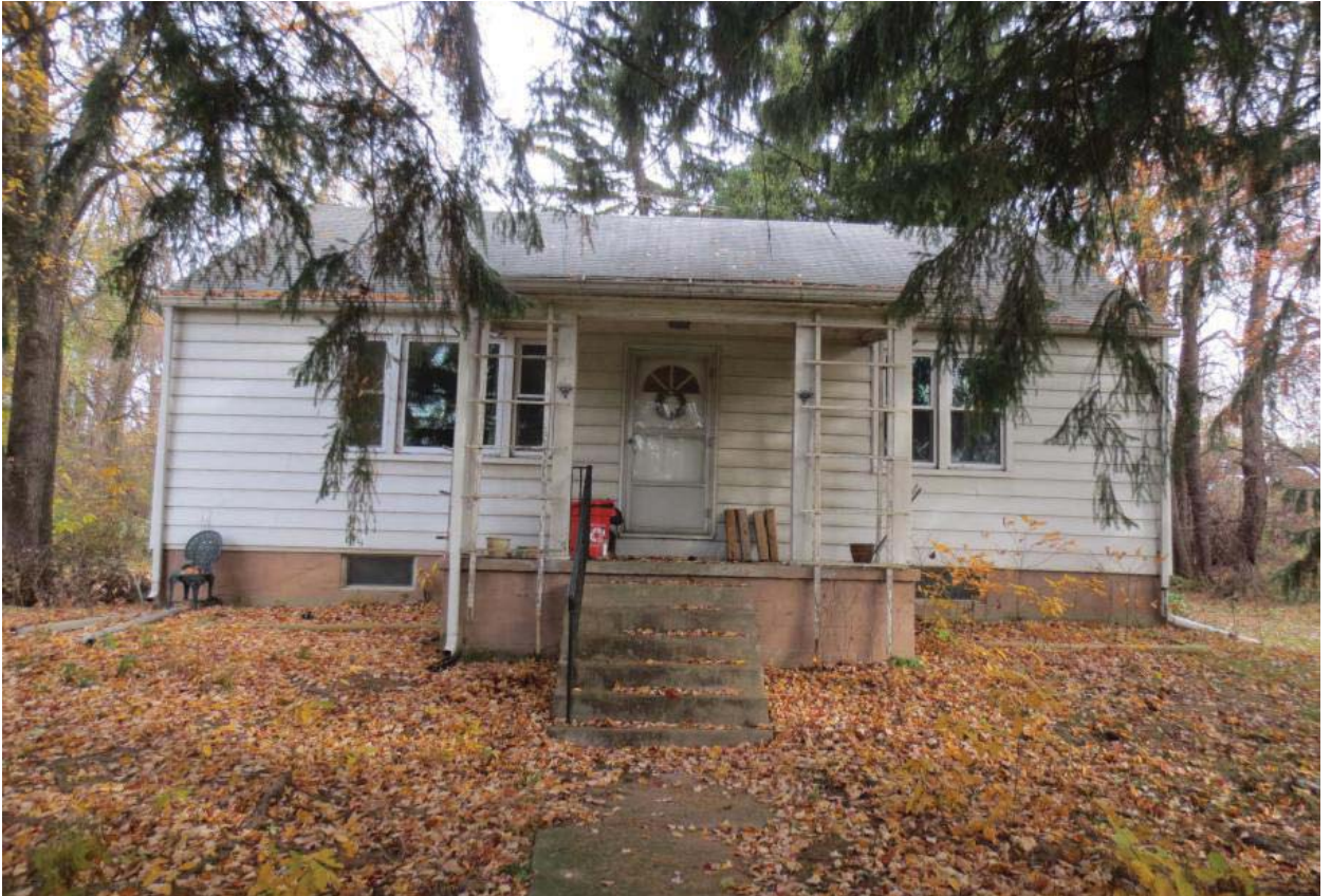
225 Rosedale Avenue - FRONT OF RESIDENCE
